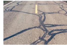
Sealed crack
