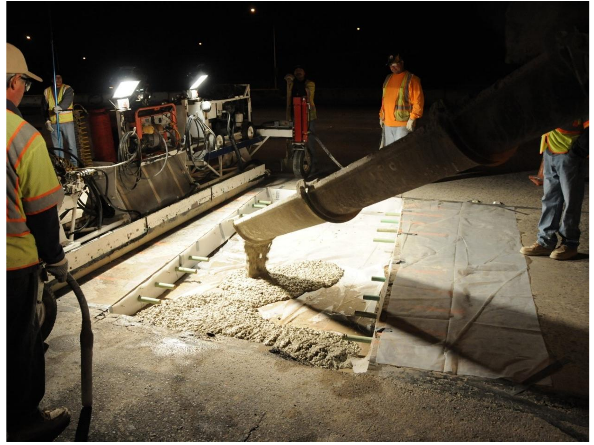
Figure 1. JPCP slabs, Caltrans [1]
