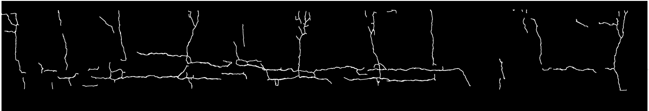
Testing Crack Map
