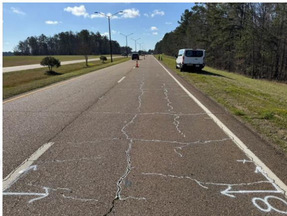
Proposed Field Labeled Crack Map
