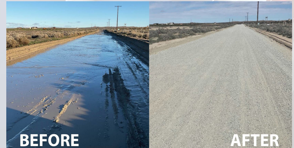
Crown reestablishment, Old El Mirage Road, San Bernardino, California
