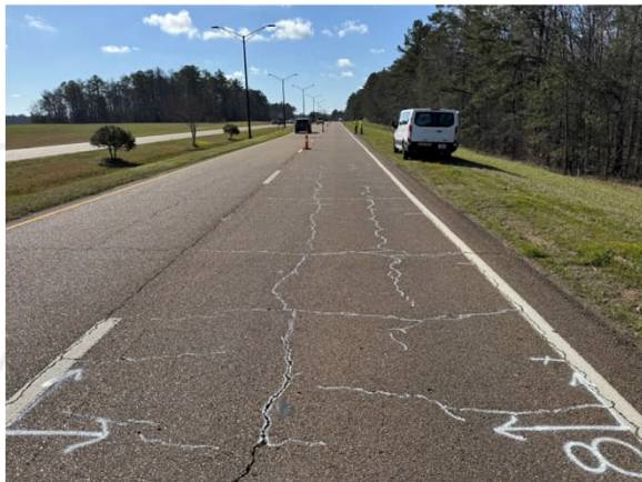
Proposed Field Labeled Crack Map
