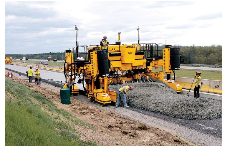
JPCP Construction using Slipform Paver
