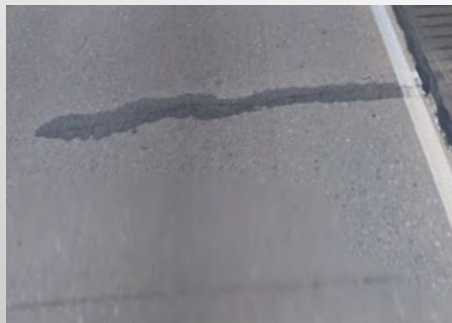
Joint and Crack Sealing
