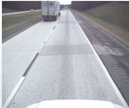
Slab Replacement (Full-depth repair)
