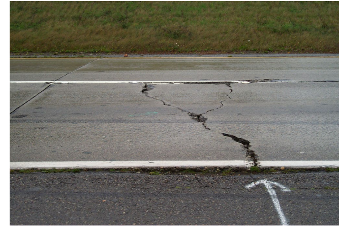
Slab cracking
