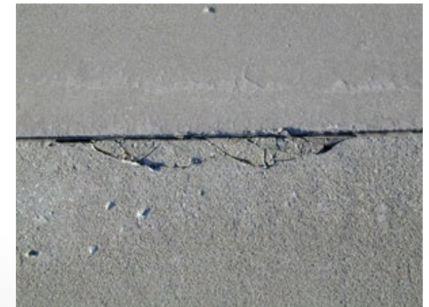
Joint spalling
