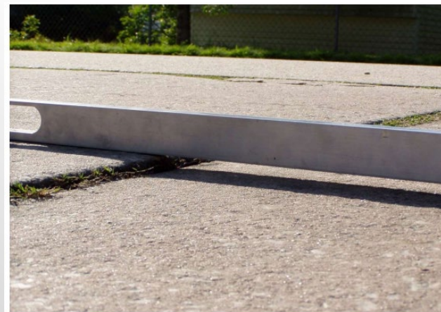
Joint faulting
