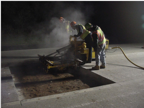
Slab Replacement (Full-depth repair)
