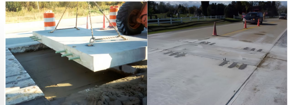
Precast Slab Replacement (Tan et al., 2024)
