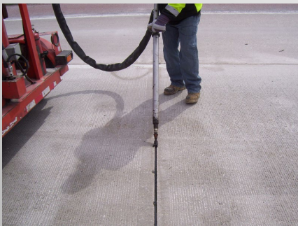
Joint and Crack Sealing
