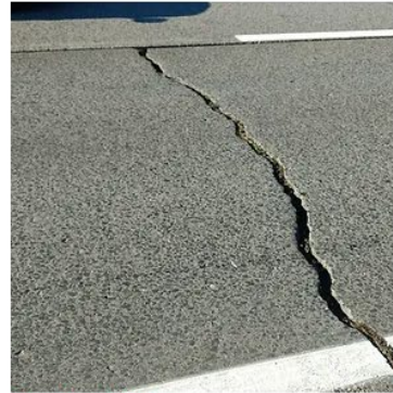
Cracked Slabs
