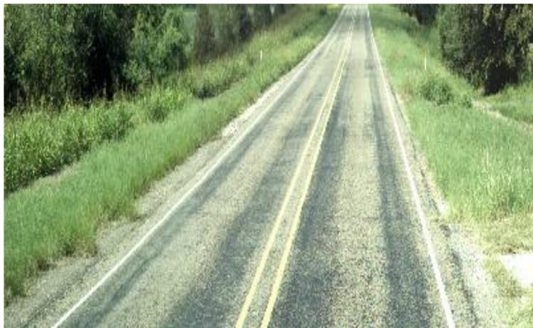
Figure 1. Example of road flushing (Highway ID: FM0020K)
