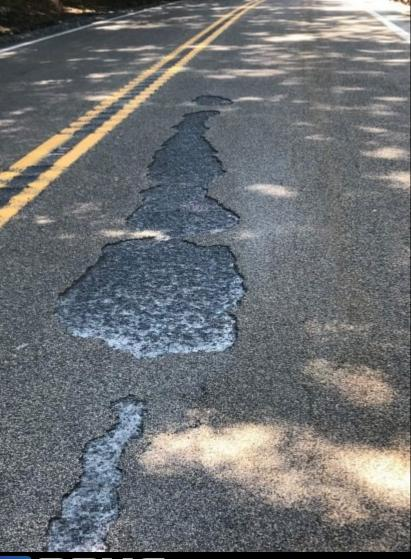
**HFST** FAILURES THAT REQUIRE **REPAIRS;** RETROACTIVE **PATCHES AND** SEALS MAY PERFORM SUB-**OPTIMALLY AT** THESE LOCATIONS
