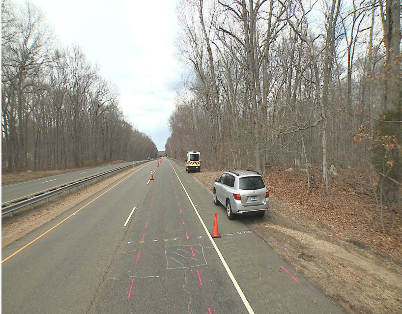
Front image of manual distress (in chalk) Section 150' to 175'
