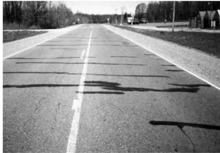
◀ Sealed cracks, a few feet apart.
