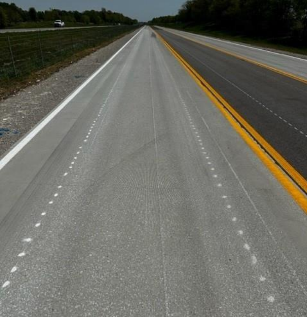
3-Smooth Finish with Diamond Grinding
